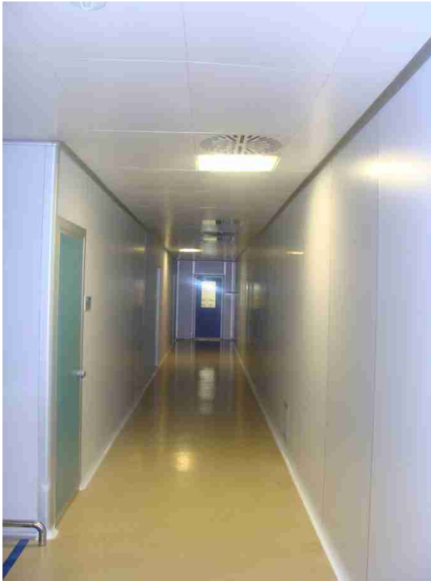
CORRIDOR, FLOOR, SIDE WALL, SUSPENDED CEILING
